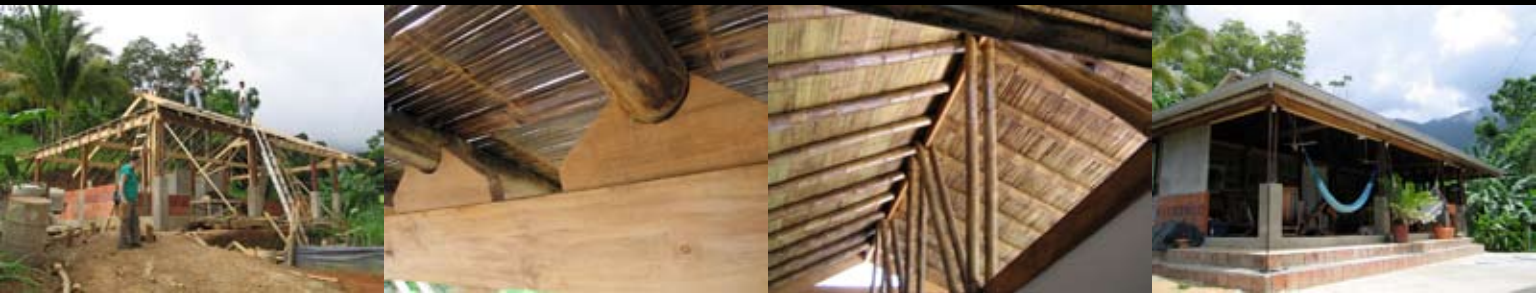
Casa Cana, small house, using bamboo as structure. In the mountain next to the project.
