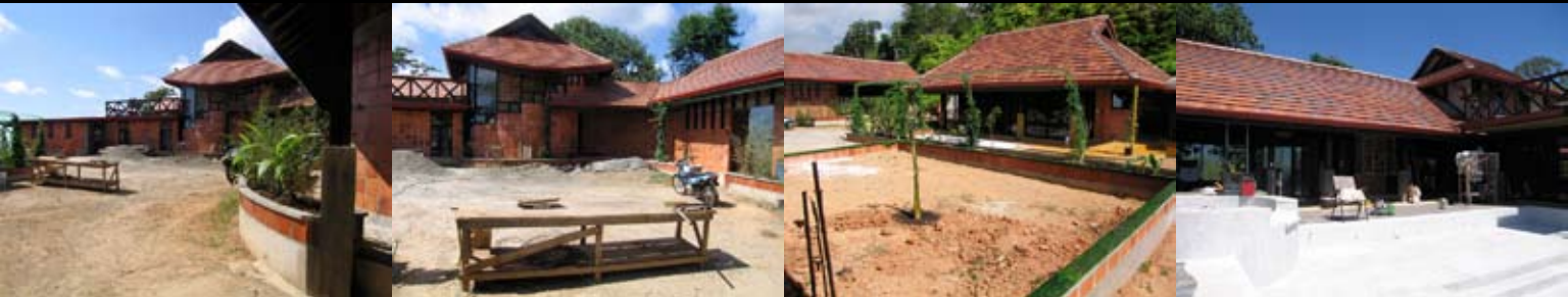
Casa Corail, a luxury house, looking over the Terraba river mouth, Osa.
